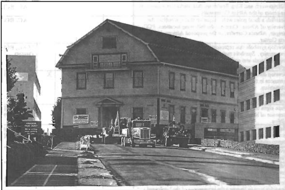
Historic Town Hall Building on N. Interstate Being Moved To New Site At Kaiser Permanente, October 13, 1990. Built by Finnish Immigrants in 1907. (Oregon Historical Society)
